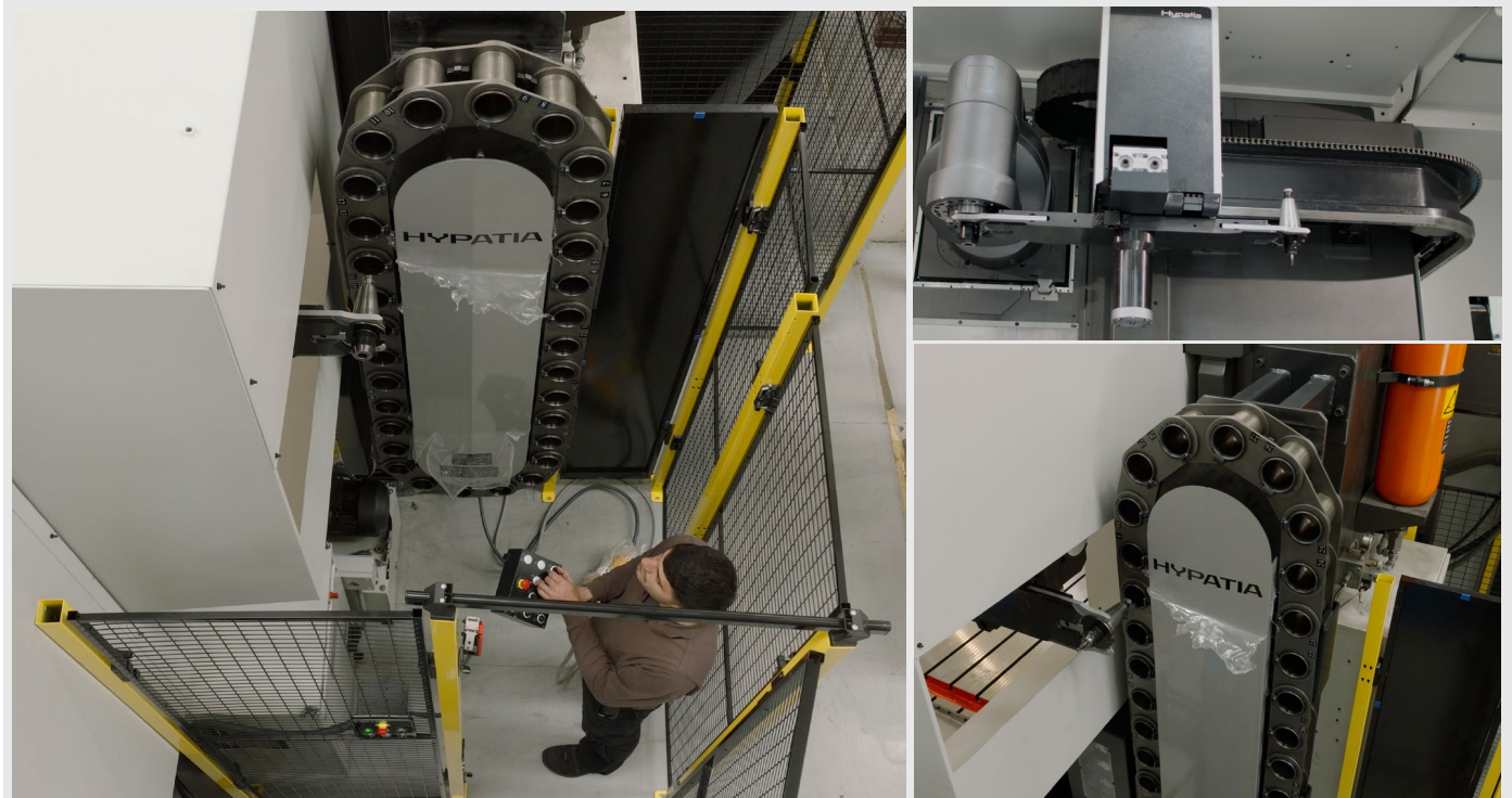
Retrofitted CORREA CF 25/25 milling machine
